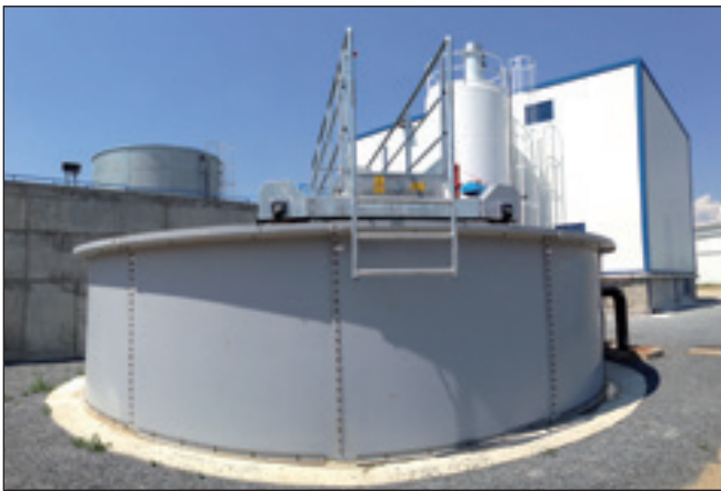
2m high W-Tank® settling tank.
