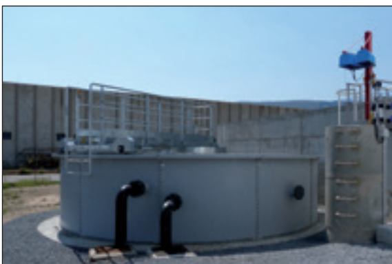
Settling tank and connections.
