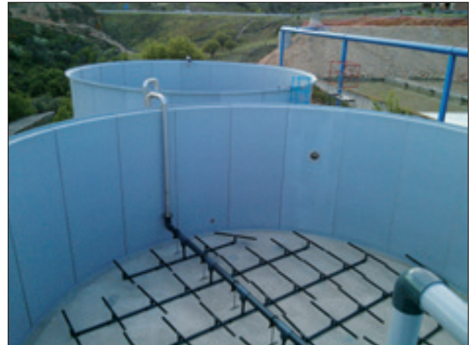
Two 5m high W-Tank® storage tanks with a diameter of 13.2m and a volume of 684m 3 .
