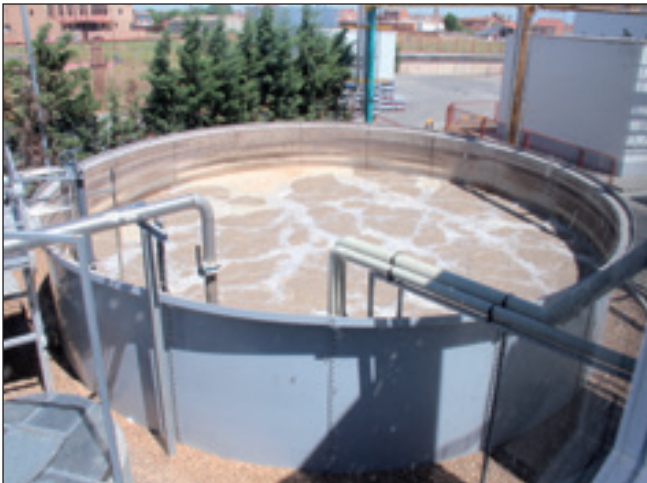
4m high W-Tank® storage tank buried 2m into the ground.
