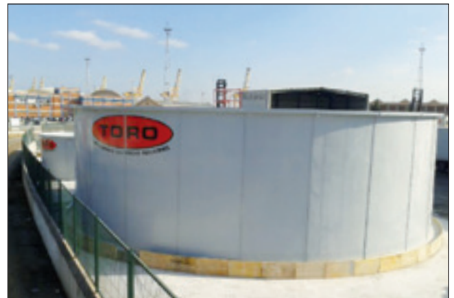
5m high W-Tank® storage tank with a volume of 993m 3 and 3m high W-Tank® storage tank with a volume of 126m 3 .
