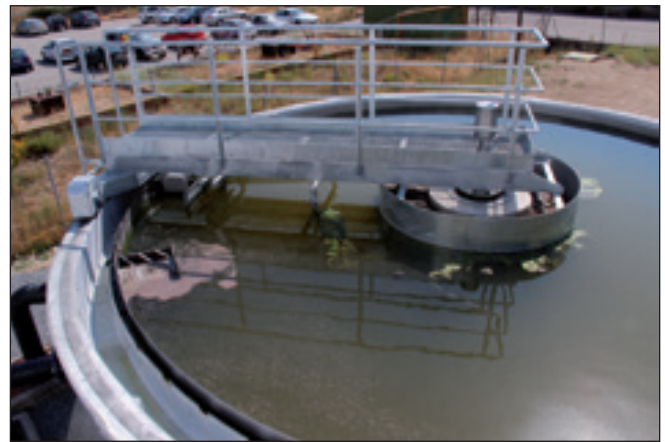
W-Tank® settling tank.
